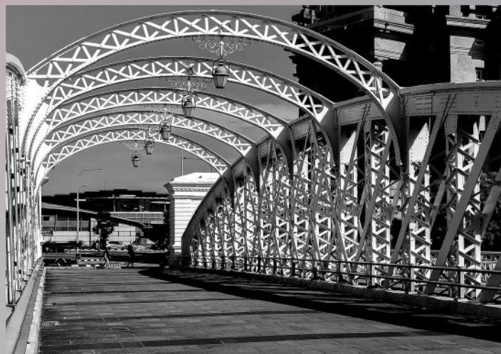
Anderson Bridge in Singapor-Olga Collet-Serret
