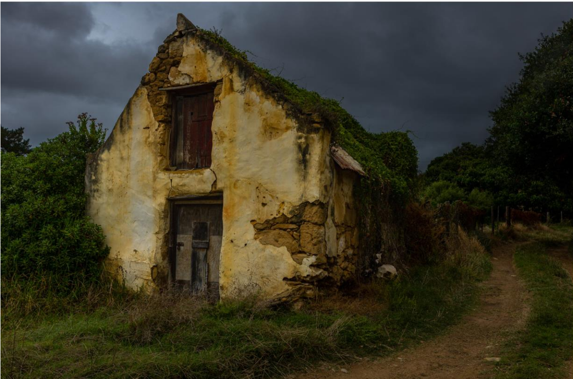
A renovators dream Giuseppe Carbonatto
